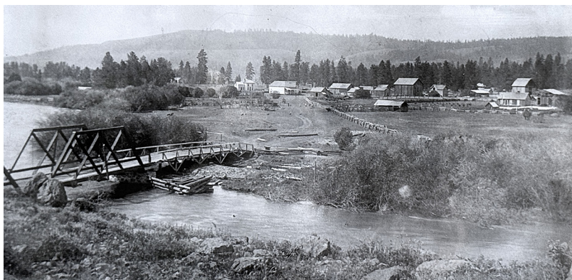
circa 1888 - Old cribbing from the first Fish Trap Bridge can be seen near the west bank of the river just below the super structure of the second Fish Trap Bridge.
